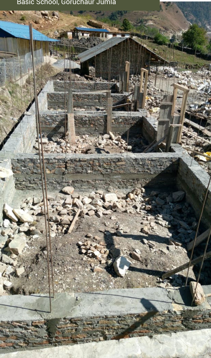
Construction Progress at Kanakasundari Basic School, Goruchaur Jumla
