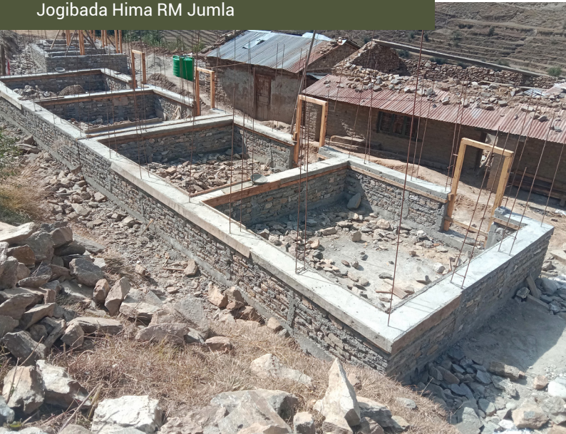
Construction Progress at Bhairab Basic School, Jogibada Hima RM Jumla
