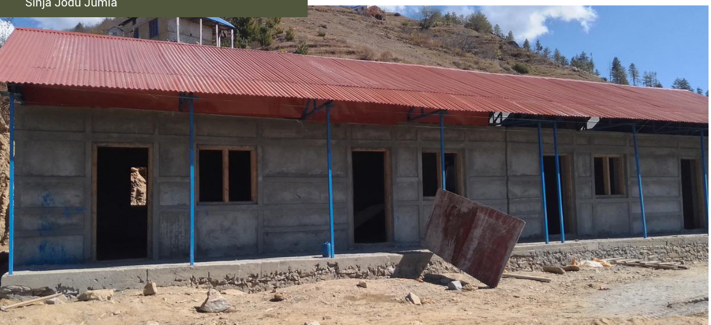
Construction Progress at Shree Secondary School, Sinja Jodu Jumla
