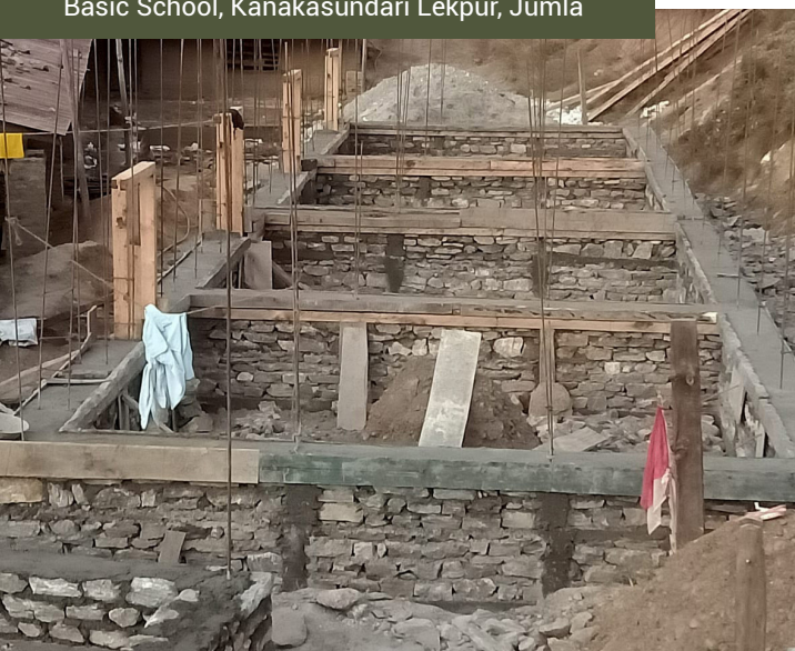
Construction Progress at Bhailepata Basic School, Kanakasundari Lekpur, Jumla
